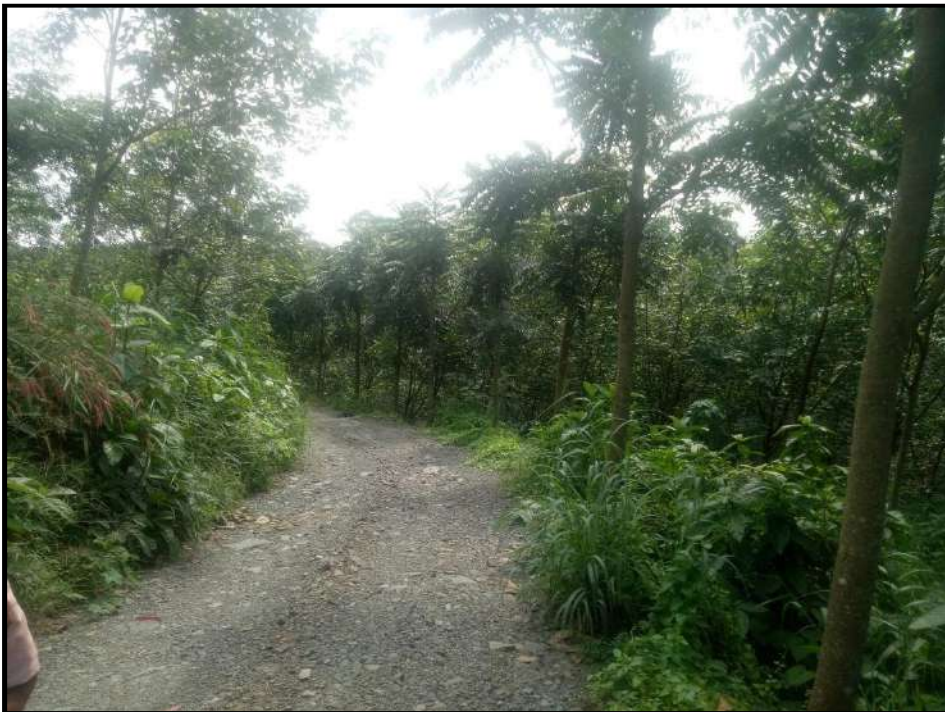
Photograph showing access road maintained by paving granite stone
